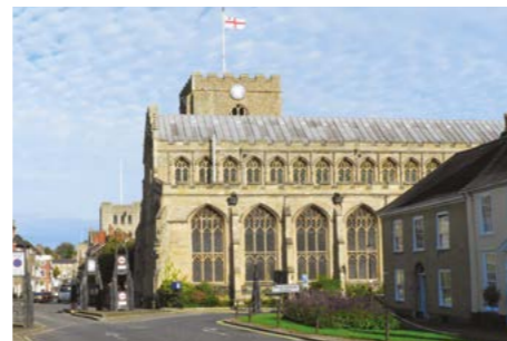
St Mary's Church and Norman Tower Photo: Richard Summers
